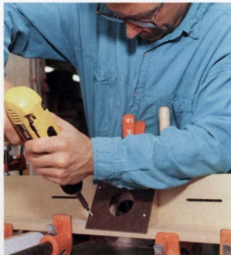
Screw dust-collection port to fence (above). Smear a bead of glue along the two triangular sidewalls. Drill holes and screw the hardboard back to them.
