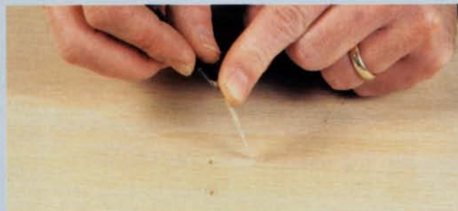
2. Cut and remove a football-shaped patch. With a sharp razor, he cuts an irregular shape around the hole to be repaired. He will fill that and the other hole with latex putty.
