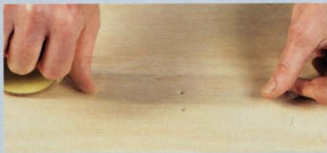
1. Cover the repair area with sealing tape. To illustrate his technique, the author drills two holes. One will be filled conventionally; the other repair will be camouflaged.
