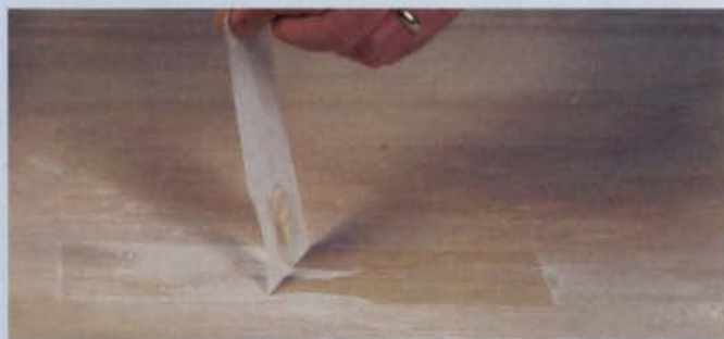
4. Remove the tape. The author sands the putty one more time to bring it flush to the surface of the wood after the tape has been peeled off.
