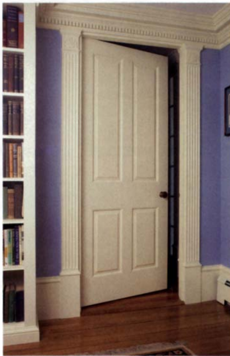
A passage door built to last—The author always dry-fits a door before final assembly (facing page) and fine-tunes the joints as required. The finished door (above) is well-suited for the site, a 150-year-old house in New England.
