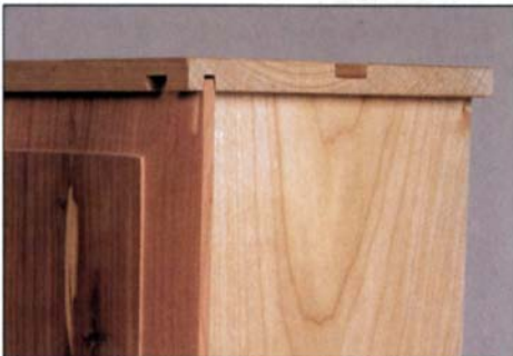
Solid raised panel in a groove
