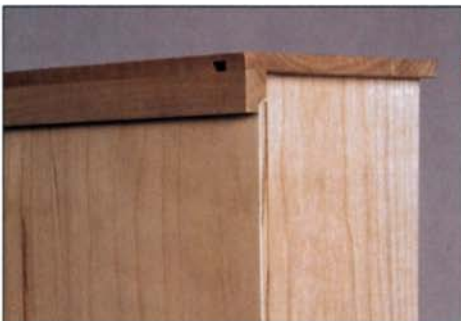
Plywood panel in a drawer slip
