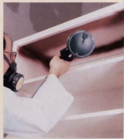
1 Spray overhead corners, and then fill in the inside top.
