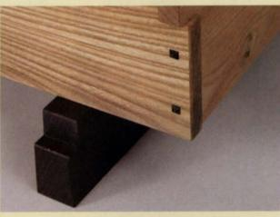
Rabbet the bottom panel to fit a 3/8-in. by 3/8-in. groove on the
