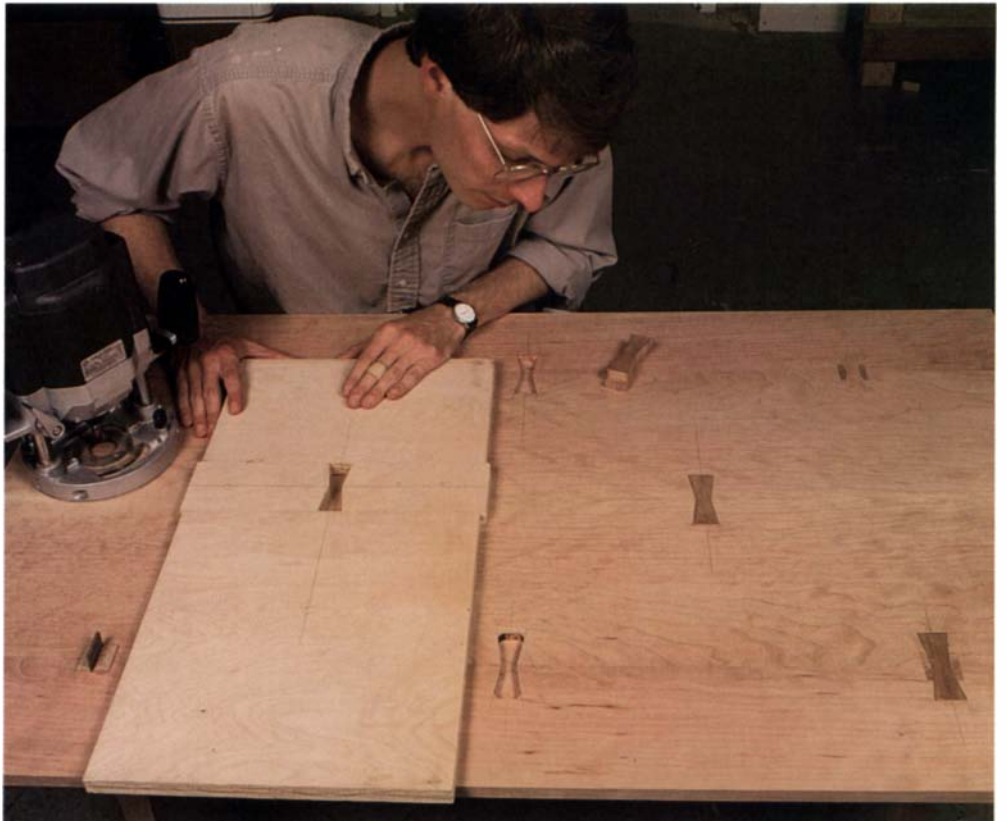
Align butterfly-mortising jig with layout lines. The rounded corners left by the router bit in the butterfly mortises are cleaned out with a chisel.
