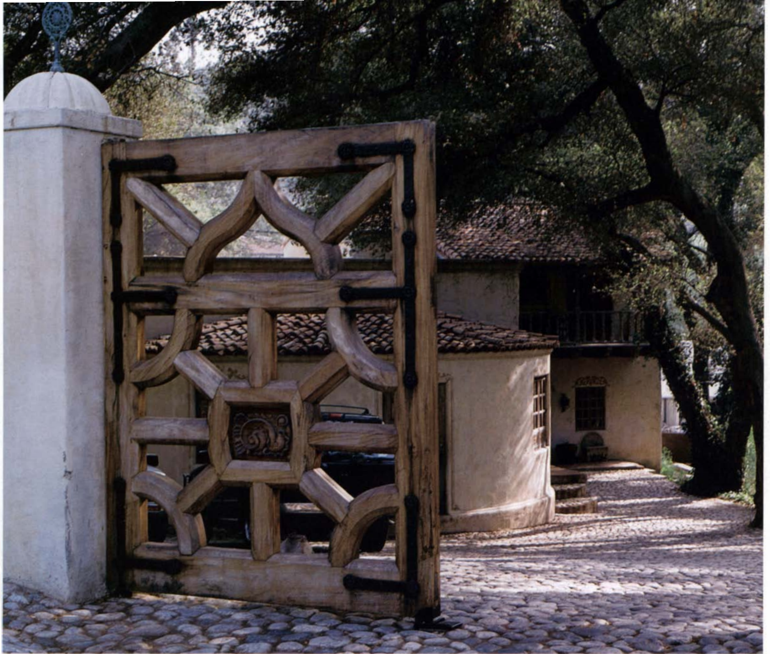
Carved Moorish gates make a dramatic entrance to Braverman's California shop. The gate has through tenons reinforced by iron hardware. Braverman carved the panel above and the door panel shown below. His wife, Kiyo, did the antique finish on both panels.
