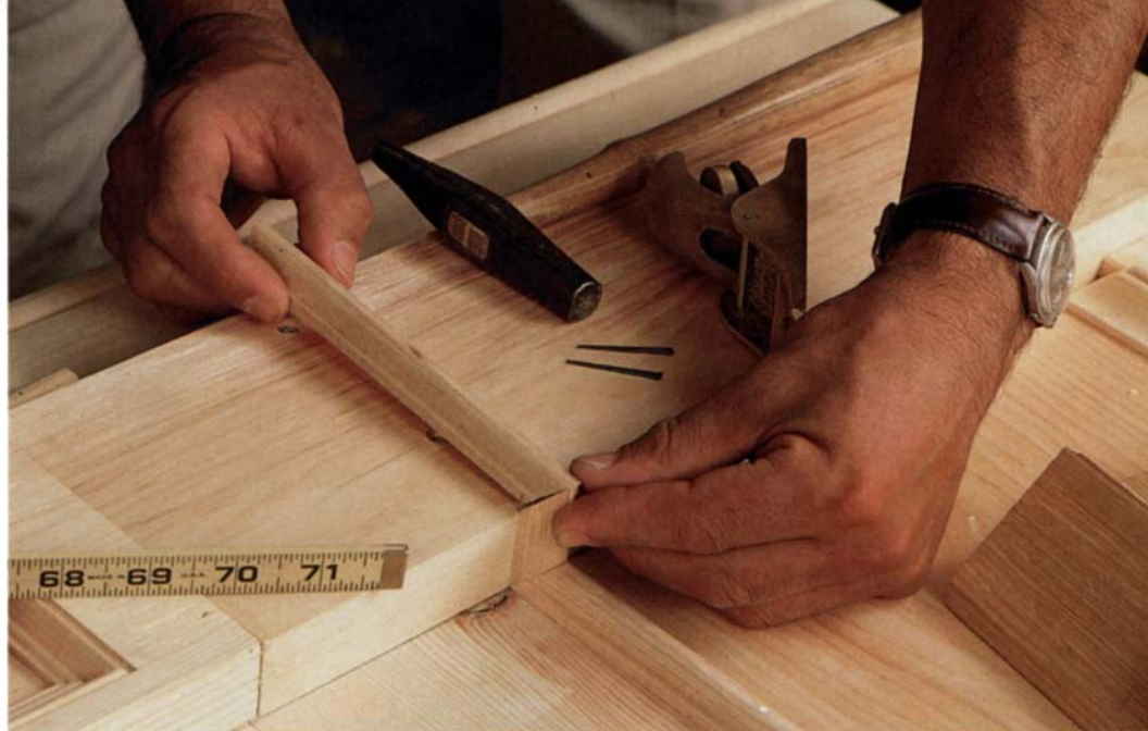
Moldings cover fasteners. Rodriguez checks his miters before gluing and nailing. This piece, about 5 in., is long enough to nail without splitting, but the smaller piece being held in place by his index finger will just be masking taped to the pilaster until the glue sets.
