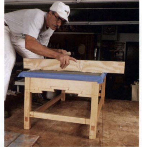
Preparing the tile bed— A notched trowel makes ribs in the wet mortar as Jordan uses the tool in the final step before setting the tiles.
