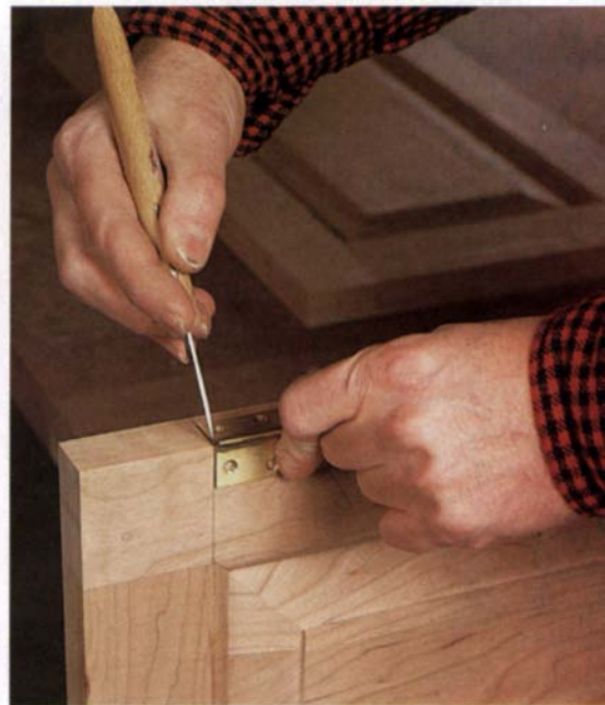
A knife is more precise than a pencil —Scribing around the hinge accurately marks its position. Darken the scribe line with a pencil to make the line easier to see when routing away the waste.
