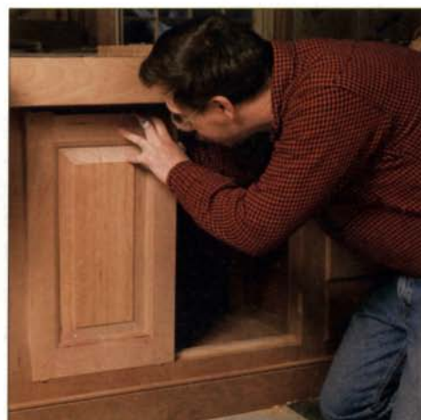
Fitting flush-mounted doors, p. 67
