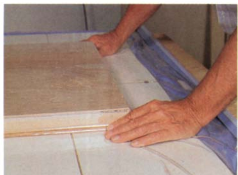
4) Eliminating air pockets
