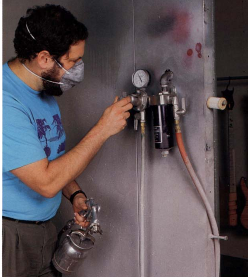
Dresdner uses a compressed-air workstation with an air filter and regulator where they are most efficient: near the end use, preventing moisture and debris in the air lines from contaminating a finish.
