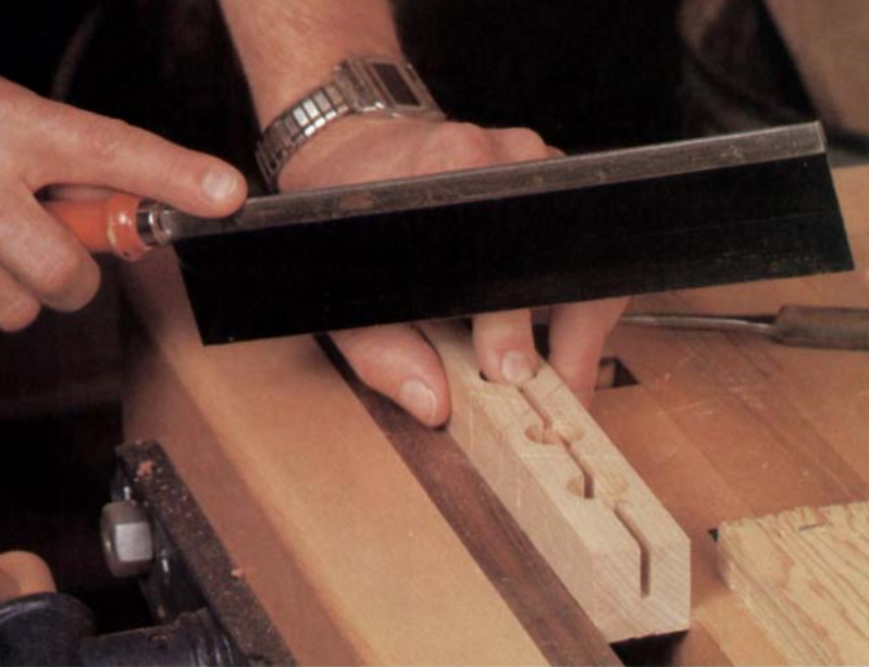
The author made two special miter boxes to cut the angles on the ends of the ribs and bars. The box for the ribs, shown here, has a few stopped holes to provide a place for a finger to hold the thin rib steady while sawing. The other box is made the same way, with a wider groove to accept the bars.
