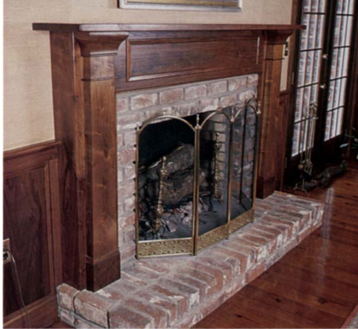
Erickson built this mantel for a fireplace on a raised hearth. The fireplace mantel extends away from the wall approximately 4 in. to accommodate the fireplace's facing bricks, which were laid proud of the wall.
