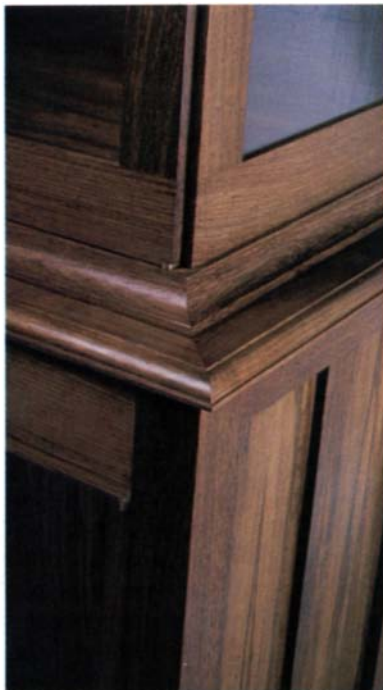
Robinson's rosewood china hutch, above, is also doweled. The lower carcass consists of a mock frame-and-panel structure doweled into a base and a solid-wood top, while the upper carcass is made of frames into which glass panes have been set. He stiffened the structure by gluing veneered panels into the solid-wood frames that form the backs of both upper and lower carcasses. Normally, panels would float freely in the frames.
