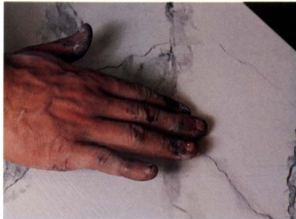
For realistic-looking marble, smudge the charcoal veins as shown above, left, to cut the contrast between the dark lines and the white base coat. Then, sponge a translucent glaze over the veins, above right, so they appear to sink into the ground coat.
