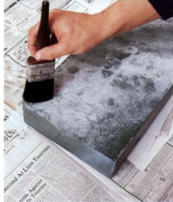
White paint—sponged on in cloudy, diagonal patterns called drifts—is applied to create the feeling of movement across the stone (above, left). A dry brush blends the drift with the green undercoat (above, right) to make the marble look more realistic.
