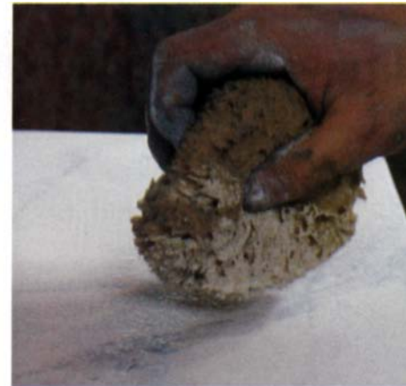
For realistic-looking marble, smudge the charcoal veins as shown above, left, to cut the contrast between the dark lines and the white base coat. Then, sponge a translucent glaze over the veins, above right, so they appear to sink into the ground coat.
