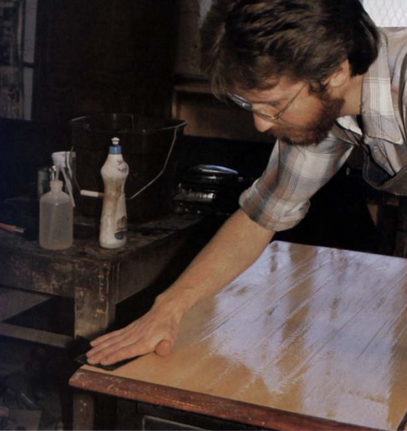
A careful rubdown with wet-or-dry sandpaper, lubricated with soapy water, dislodges dust nits and levels the lacquer film. Johnson completes the job with 4/0 steel wool lubricated with a commercial steel wool lubricant.
