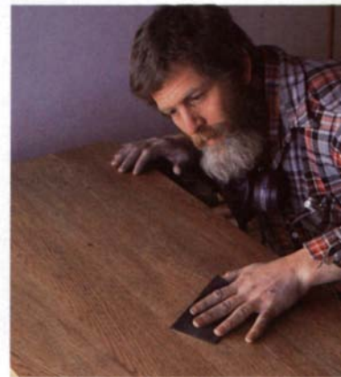
Shaw sprays catalyzed lacquer just like regular lacquer, with long, even, overlapping strokes, above. A double-cone, organic vapor respirator and fans or other forced ventilation are mandatory. Finishing the finish is the most time-consuming part of the job. To ensure a rich, smooth finish, each coat must be rubbed out with fine wet/dry paper. To check his work, right, Shaw examines the finish closely from a low angle where light reveals any defects.
