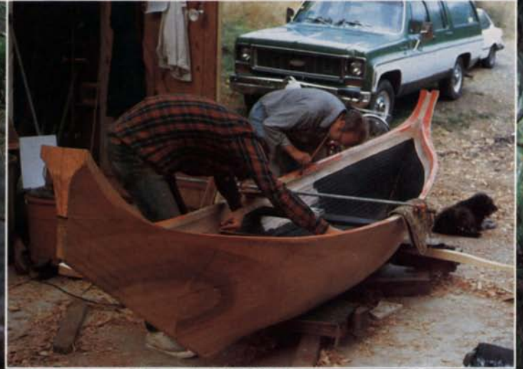
Granum's dugout canoe, based on a traditional Northwest Indian design, is carved from a single red cedar log, then steam-bent to its final shape. Shaping is done with a variety of adzes (top, left and center). The wood bridge prevents warping during carving. Hot rocks heat the water for steam bending (top right), and 2x6 spreaders almost double the width of the log. Granum painted the finished canoe with his own grizzly bear designs.
