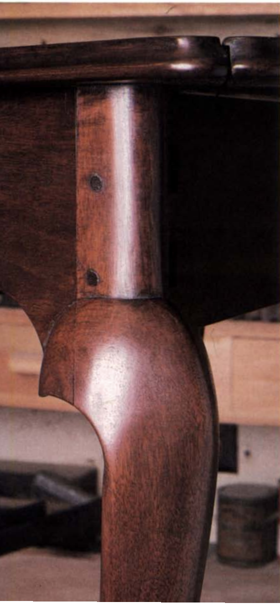
A look at the table's back corner (left) shows how the knee and post have been shaped to conform to the 45° angle. The hinged back leg nests as shown at right; note in the drawing on the facing page that both legs are oriented in the same direction. Below, Landon demonstrates the setup for starting an angled mortise. He supports the corner post in a V-block, and presses the leg against his forearm for extra control. Paring the tenon's angled shoulders is shown at right below. The first step is to bandsaw close to scribed layout lines. Then finish up with a chisel and a 45° guide block.
