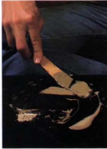
To make a wood filler, use a hera (wooden spatula) to mix pulverized stone powder with water, then work in a small amount of lacquer until the paste can be smeared easily.
