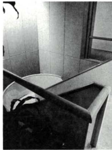
O'Hearn's biggest challenge is understanding the architect's intent and then transforming arcane drawings into woodwork, as shown here. Large-section moldings, which trim the top of the stair's rail, are a main staple of most millwork shops.
