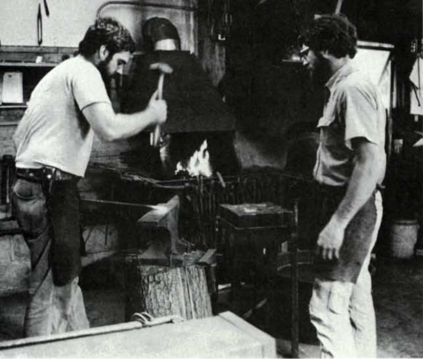
The basic tools of the blacksmith—fire, hammer and anvil—have remained unchanged for hundreds of years, and the smith's products are similar to those made by his colonial forebears. Wrought thumb-latches and H-hinge by Woodbury Blacksmith and Forge Co., right, show the distinctively varied profiles left by the process—no two are identical, and the marks left by the smith's hammer and anvil are evident.
