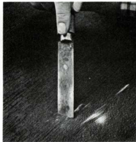
Clean and reheat the knife and drag it bevel-side down to smooth the resin to the surrounding surface.
