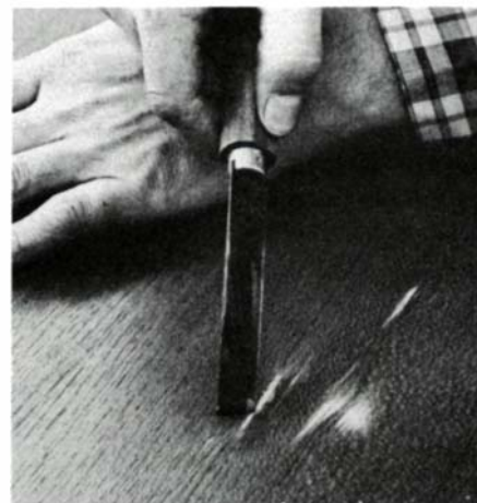
To fill a scratch, apply a bead of resin to the heel of the hot knife. Then push the resin-coated heel into the scratch and rock it gently to distribute the resin.
