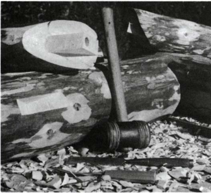
Gouges are used to finish shaping the scribed shoulder of a brace log, above. The hole, which will receive the all-thread, was bored the entire length of the log before the tenon was cut. Below, a finished joint.
