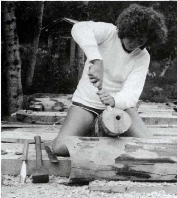
Gouges are used to finish shaping the scribed shoulder of a brace log, above. The hole, which will receive the all-thread, was bored the entire length of the log before the tenon was cut. Below, a finished joint.
