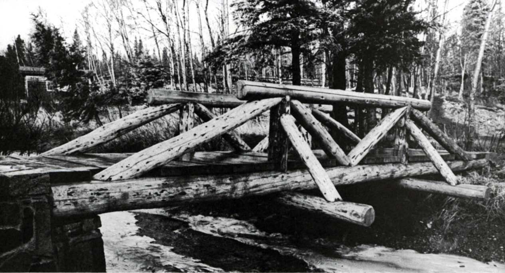
Scribed mortise-and-tenon joinery in this 29-ft. trussed log bridge make all its parts securely interdependent.
