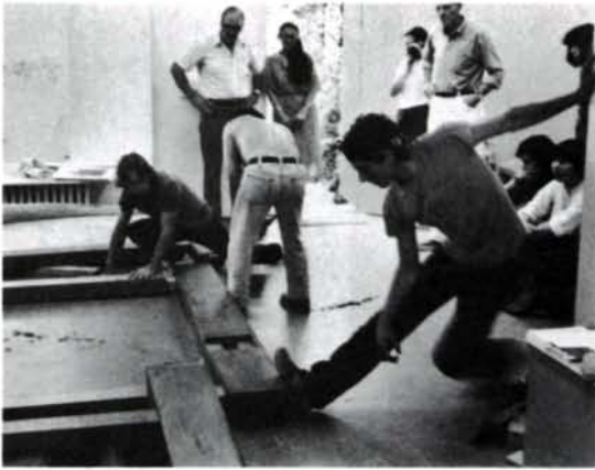
Odate (shirtless) commands one of the top members into place, above. More help was required to upright the 3-in. thick white oak flitch mounted in mortise-and-tenon timber frame, right. Screen frame, center right, was drawn to flitch frame with clamps.
