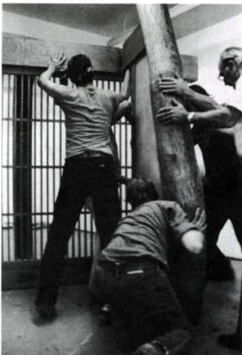
Cement wing with cherry log is slid into place.
