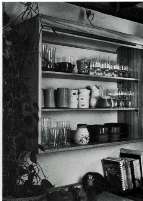
Tambours in the Weed kitchen allow cabinets (all made of black willow) to remain open without swinging doors on which to bump your head or to obstruct access. Weed says this design requires no more work to make than a set of frame-and-panel doors. Right, tambour curtain disappears behind faceboard and false back, painted white. A stiffener strip neatens the top edge of the false back. Cabinet is deep enough for stacks of 10-in. plates.
