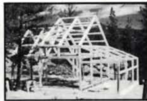
A GUIDE TO HOUSE RAISING
