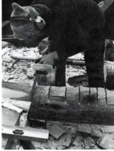
Two-person timber carrier and trolley, left, bring log to where it can be scored with a symmetrically beveled ax, hand saw or chain saw, center. Then log is rotated 30° and waste wood chopped with a symmetrically beveled ax to within 3/8 in. of the chalkline, right.
