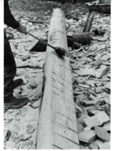
Two-person timber carrier and trolley, left, bring log to where it can be scored with a symmetrically beveled ax, hand saw or chain saw, center. Then log is rotated 30° and waste wood chopped with a symmetrically beveled ax to within 3/8 in. of the chalkline, right.
