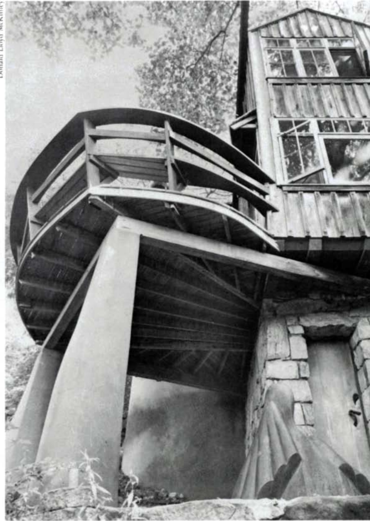
The south face of the Esherick studio and home includes the door that opens onto the coat room (shown behind the staircase, p. 54). Above is the dining area, and above that a bedroom. The foundation is limestone, the siding roughsawn oak, and the deck cedar and fir, supported by stone and plastered pillars.
