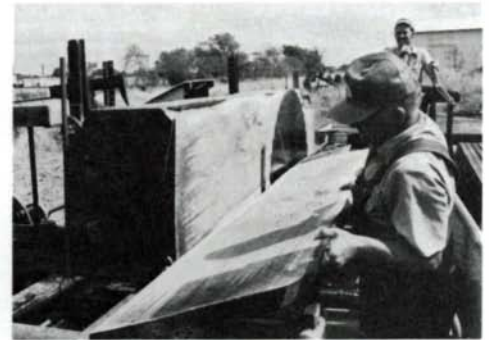
Sawyer and off-bearer are a team. Here board is held away from contact with trailing edge of blade and pulled down as carriage is giggered.
