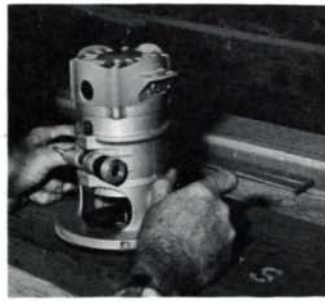
Left, Wilbur traces image cast by overhead projector directly onto the wood, then routs out sample letters, above. The heels of the hands rest firmly on the wood to guide the router through each letter. Some of his finished signs are shown at right.
