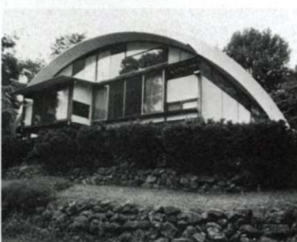
The Conoid Studio, inside and out, and some of the wood standing around the walls. The arching roof is a thin, undulating shell of reinforced concrete, which flattens out to a line at the rear of the structure. The building mostly serves as a showroom and as Nakashima's private office and studio. The raised platform at the right of the interior view is equipped for the traditional Japanese tea ceremony.
