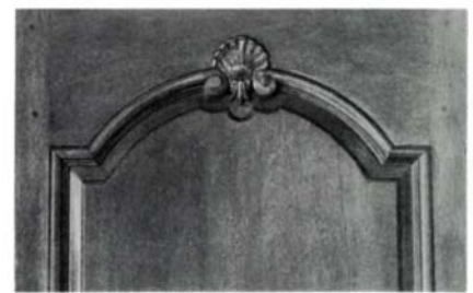
Mahogany door to Panayi's shop has arched panel and shell carving. Two square tapered pegs driven through each mortise cheek lock the tenon in place.
