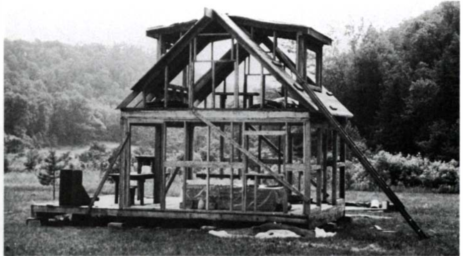
Left, concrete block foundation, built on concrete footings, supports solid 6x6 girder and 2x6 oak joists. Frame, above, requires diagonal bracing until particle-board sheathing is nailed on.
