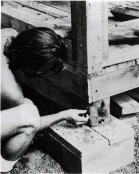
Left, concrete block foundation, built on concrete footings, supports solid 6x6 girder and 2x6 oak joists. Frame, above, requires diagonal bracing until particle-board sheathing is nailed on.
