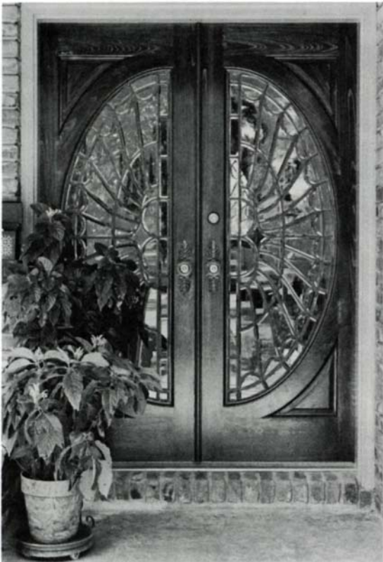
Michel Panayi of Houston, Tex., runs a two-man shop that specializes in solid wood frame-and-panel doors. This door, of cypress, was designed around the customer's glass. Panayi favors cypress for exterior doors because it is both weather-resistant and strong.
