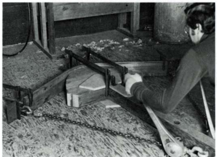
Cross-bow mold is made from telephone-pole crossarms and fitted with one-ton chain hoists. Center clamp at base of mold and two more clamps hold wood firmly in place as hoists pull it around.
