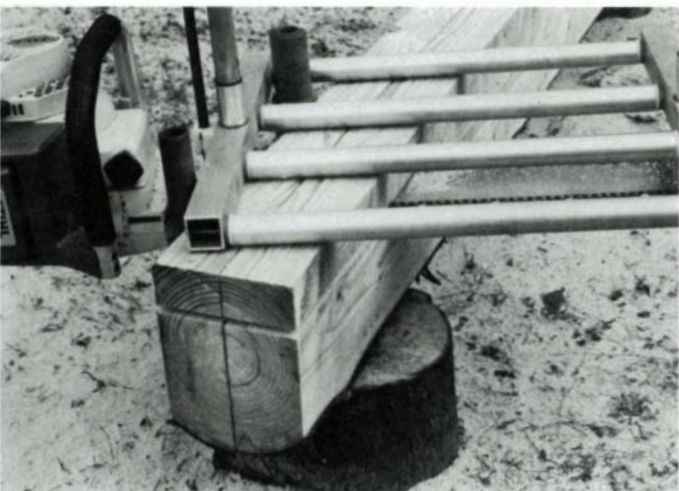
After 90° rotation of log and first cut on top (with slabbing rail), log is square on three sides. Now groups of 2x4's can be sliced off, and separated later. By changing the mill settings, most construction lumber can be cut easily.
