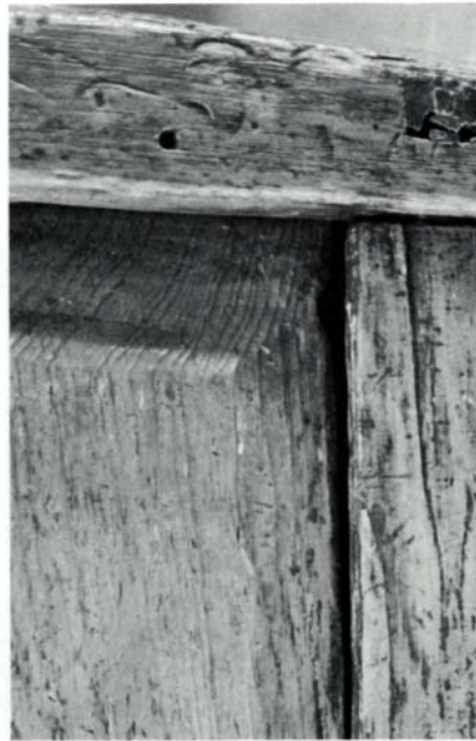
Low humidity has caused the wood to shrink to such an extent that the edge of the panel is exposed. At right, butterfly keys on a mitered joint. The middle key was inaccurately laid and required the use of filler.
