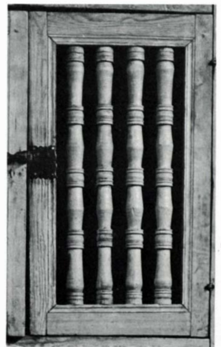
A multiple-panel door in pine. The panels were beveled with a gouge. The use of spindles (below, right) in the central section of this trastero door accommodates wood movement and also allows the contents of the cupboard to be viewed.
