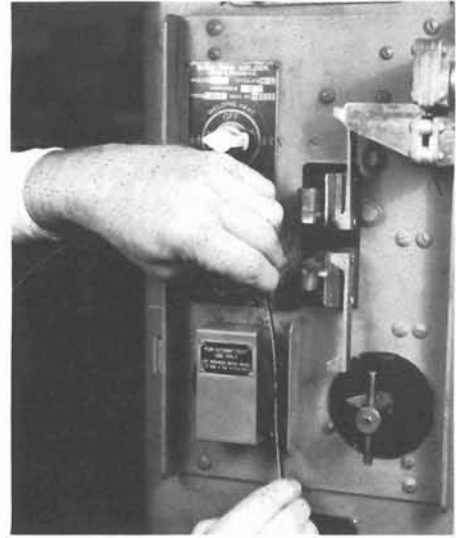
9-62. The bead or welding flash is carefully removed on the build-in grinding wheel.
