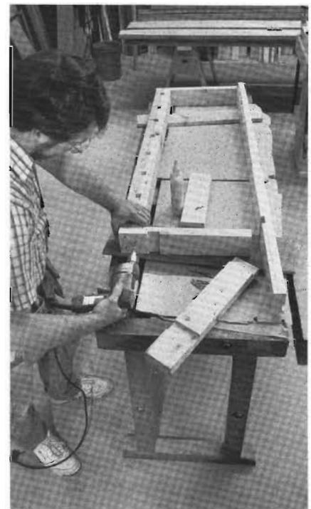
2-4 The top frame includes the bench dog assembly. I use glue and 2½-in. drywall screws to join all the parts together.
