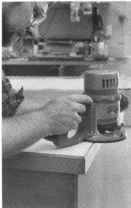
6-13 With a chamfering bit in the router, I give the sides and front of the countertop their finished edge treatment.
