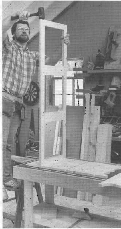
11-3 Glue and nail the lower frame and plywood shelves into their dados, one side at a time.
