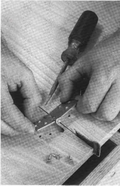
3-13 The pin of the drop-leaf hinge fits in a 1/4-in.-wide groove cut in the underside of the top's center section. A piece of sandpaper, temporarily wedged in the drop-leaf joint, provides 1/16 in. of clearance between the pieces when the hinge is first screwed to the table.
