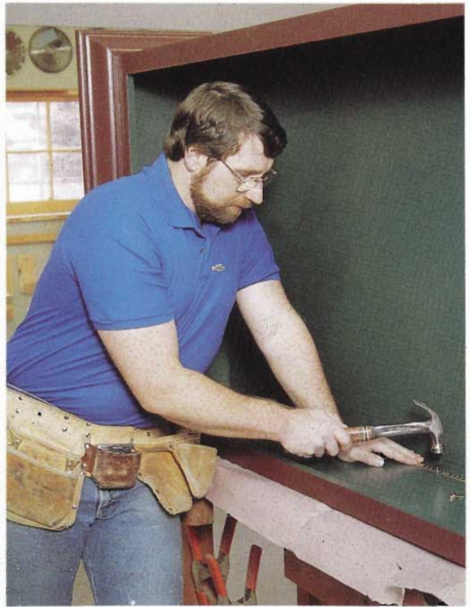
8-11 Install the shelving standards after the case has received its finish. Before nailing the standards in their dadoes, make sure that matching holes are level.
