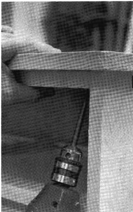
9-13 Attach the top by driving 1 1 / 4 -in. drywall screws through the top frame from inside the chest.
