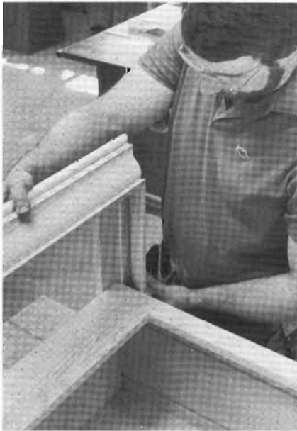
8-9 The completed head casing fits snugly, but can be taken off by removing a few screws.
