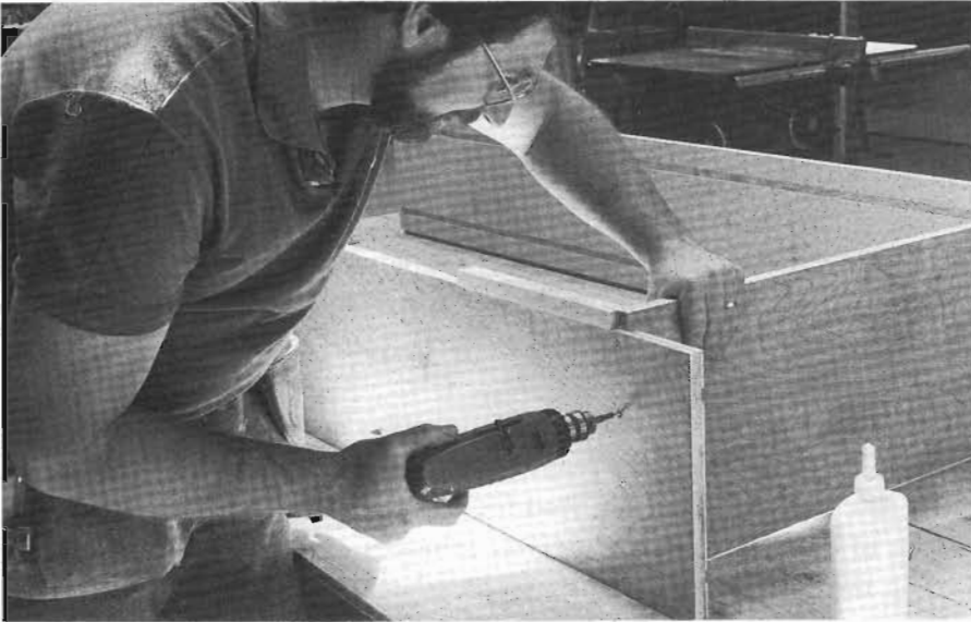
8-4 The bottom shelf is glued and screwed into dadoed sides. Before driving screws, make sure that the bottom's front edge extends 3/4 in. beyond the sides' front edges.
