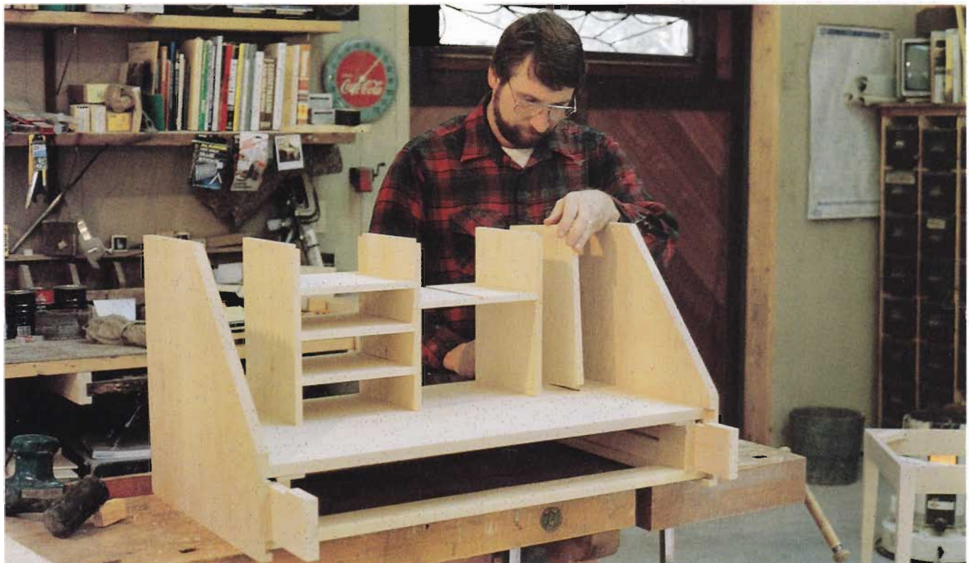
12-11 Vertical compartment dividers are glued into their dados in the work surface. The desk top will then be glued into the sides and over the vertical dividers.
