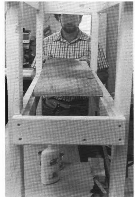
2-7 With the frame right side up, slide the lower plywood shelf into its rabbeted frame and screw it down.
