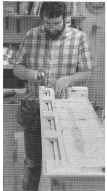
11-16 Install angled blocks to keep the top edge of the molding even and strengthen the upper part of the cornice. Fasten the blocks to the top edge of the angled cleat and to the back of the molding.
