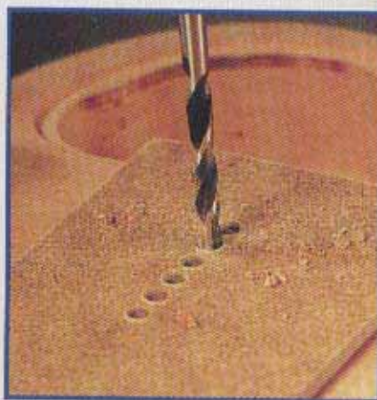
33 Drilling ferrule holes using template
