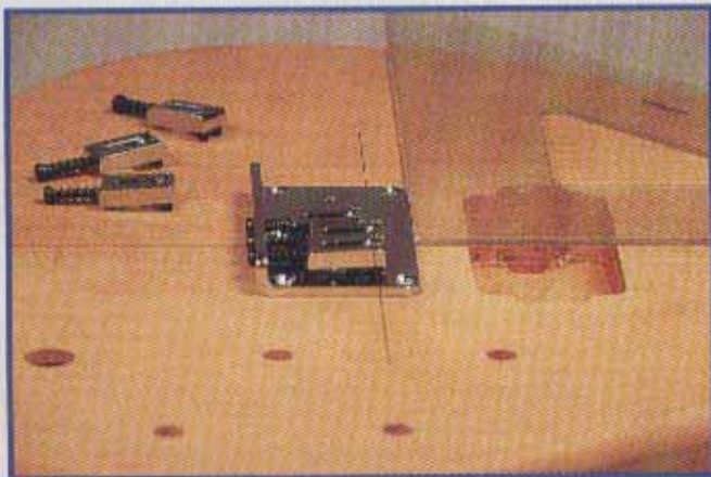
27 Placing and squaring the bridge
