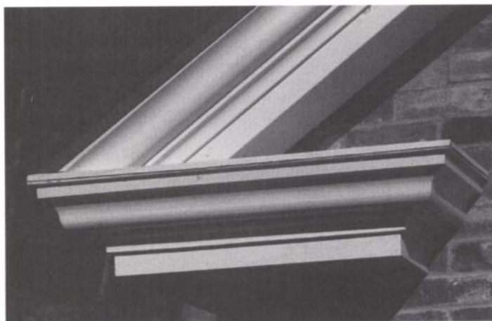
The completed cornice on the author's shop was made in two pieces and shaped entirely with molding planes.
